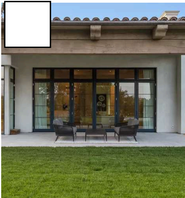
Broom Finish Concrete
